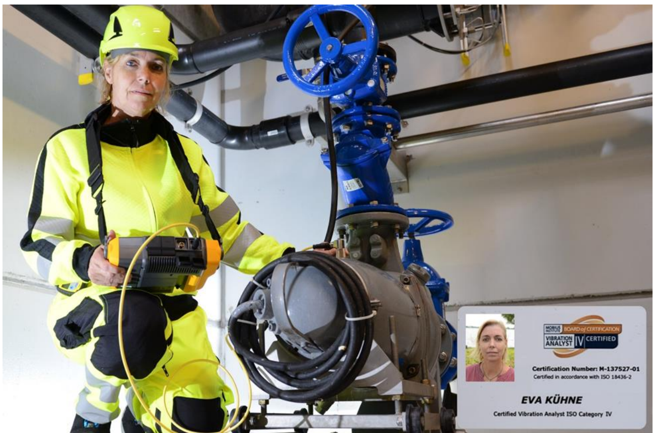
Figure 59: Route-based monitoring on a dry-installed wastewater pump.
