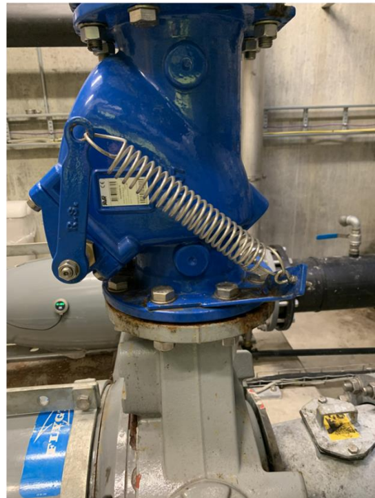
Figure 23: Pictures from an application. Picture to the left illustrates the broken non-return valve spring, and the picture to the right shows the valve with a new inserted spring.
