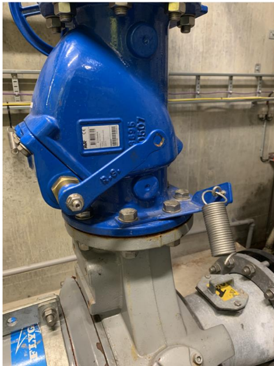
Figure 23: Pictures from an application. Picture to the left illustrates the broken non-return valve spring, and the picture to the right shows the valve with a new inserted spring.
